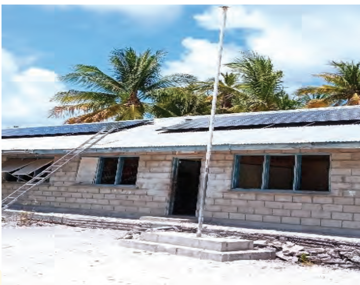
Solarisation of Nawai Junior Secondary School on Tamana Island, Kiribati
